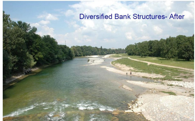
Diversified Bank Structures- After
