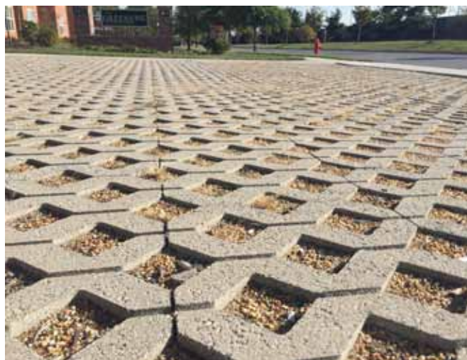
Figure 5. Concrete grid pavers are a good option to reduce runoff from parking lots
