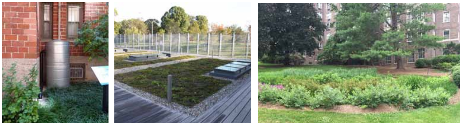
Figure 13. Three options for managing rooftop runoff in Washington, DC: 1) rain barrel, 2) green roof, and 3) disconnected downspout directed to a rain garden
