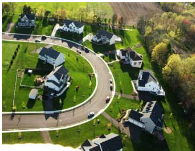
Figure 9. The roadway comprises a significant portion of impervious cover in this neighborhood, compared to sidewalks (Photo credit: Dorothy Cappiella)
