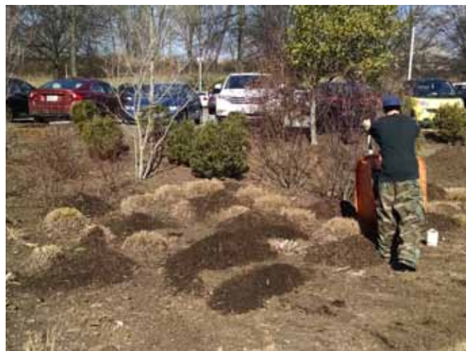
Figure 17. Mulch replacement is one activity that may be included in a maintenance agreement for stormwater practices such as bioretention.
