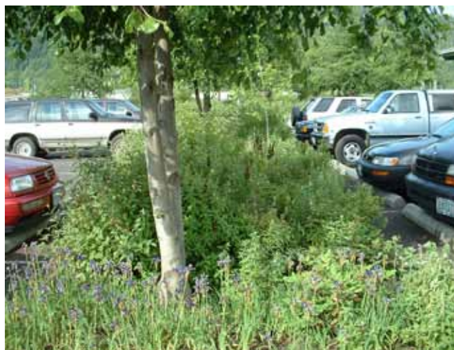
Figure 6. This landscape area is designed to accept and treat stormwater runoff in this Portland, OR parking lot
